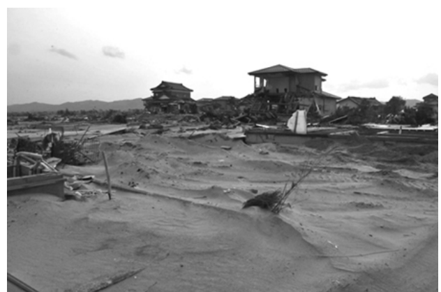
Fig.5 House lots covered with sand after the tsunami in Yamamoto Town, Miyagi Prefecture (photographed by the author).
