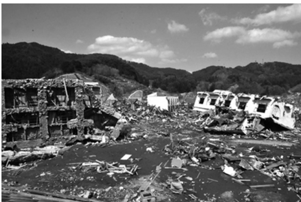
Fig.9 Appalling damage to Shinminatomachi neighborhood (photographed by the author).
