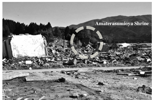
Fig.4 Amaterasumioya Shrine in Rikuzentakata City escaping collapse (photographed by the author).
